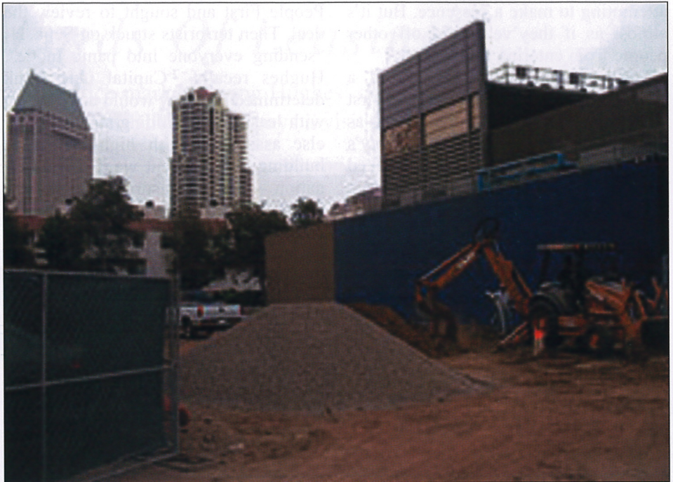
Site preparation has already begun for the 23-story Broadway 655
