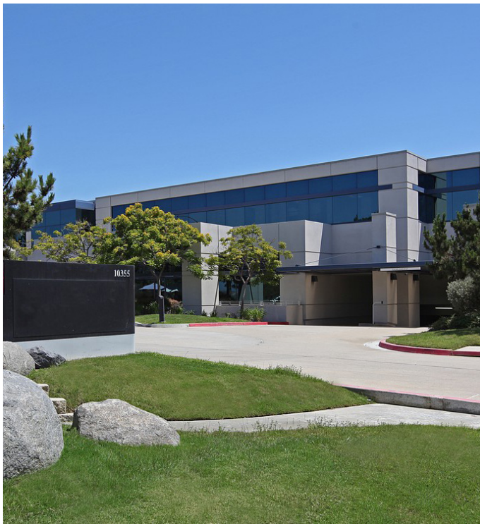
HCP's new life science facility on Science Center Drive offers options for smaller tenants.
